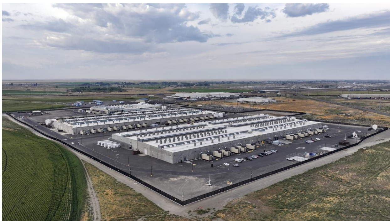
Figure 30: Amazon Web Services Data Center, Boardman Oregon, 2024 4
